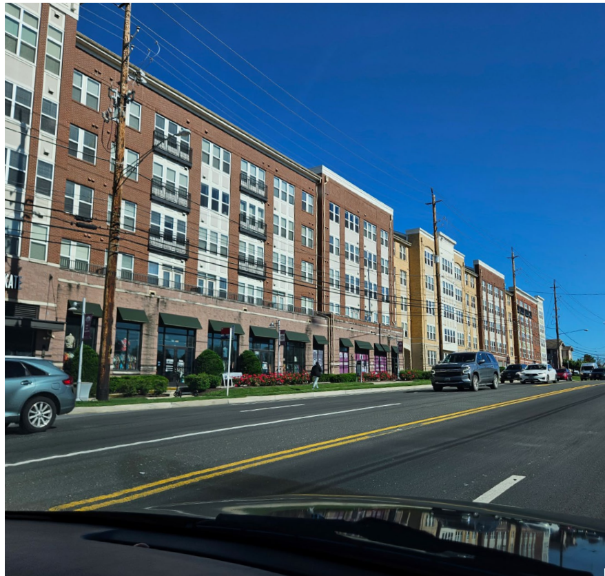
Existing Conditions Baltimore Avenue
