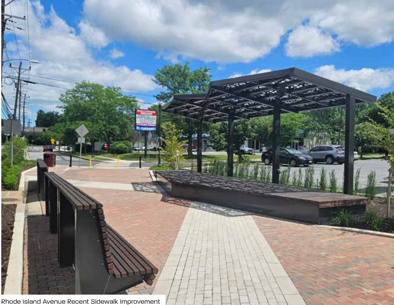
Rhode Island Avenue Recent Sidewalk Improvement
