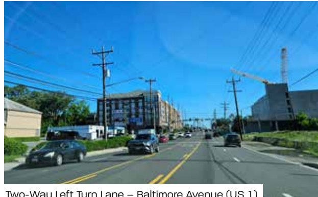
Two-Way Left Turn Lane – Baltimore Avenue (US 1)
