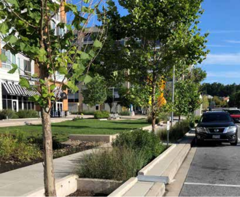
The Metropolitan, Columbia, MD Street Tree Rainwater Planters and Artful Bioretention
