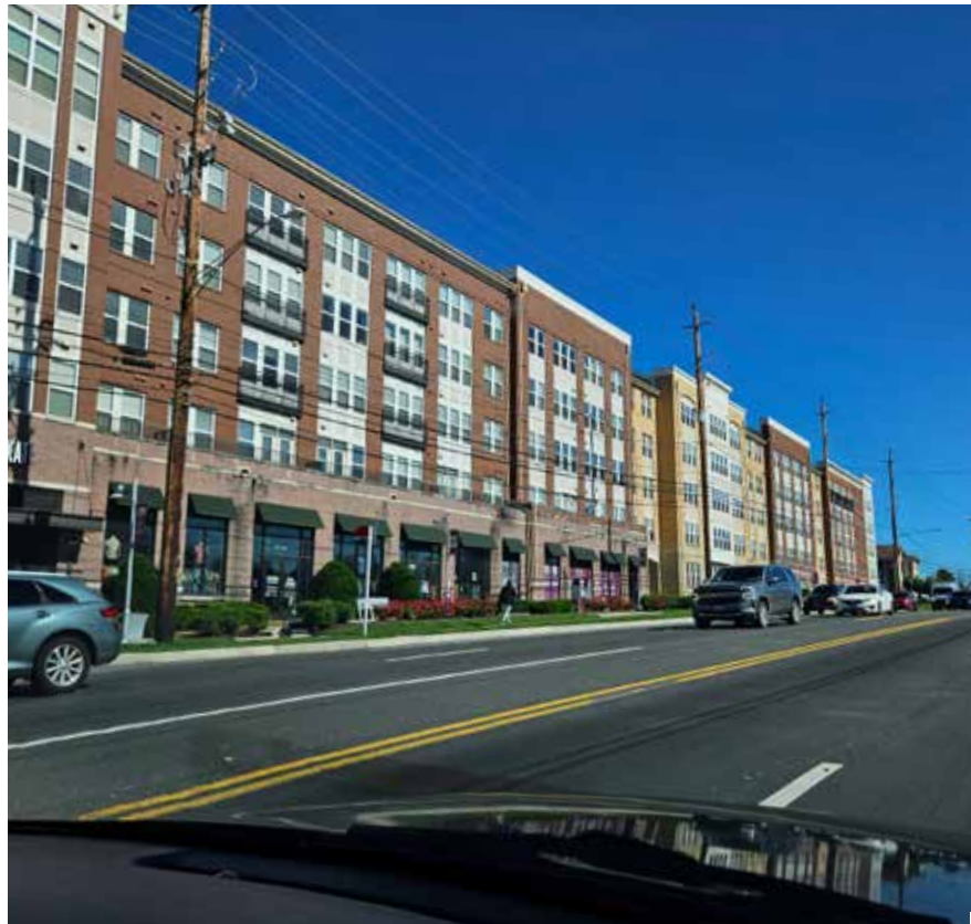
Existing Conditions Baltimore Avenue
