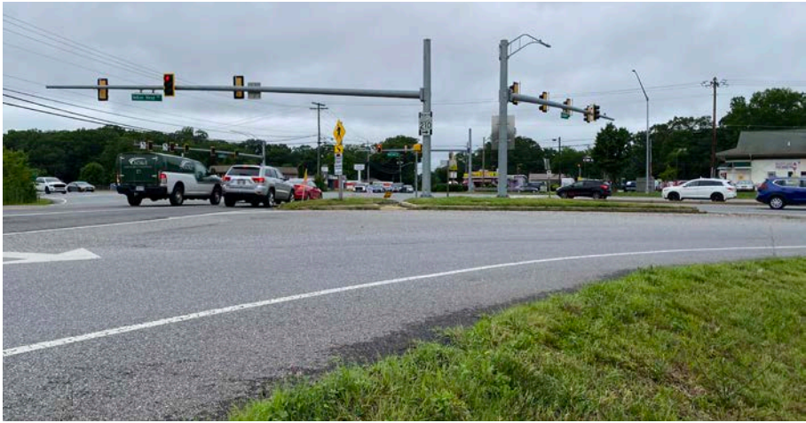
Right turn slip lane at intersection of MD 210 and MD 373 (Livingston Road)
