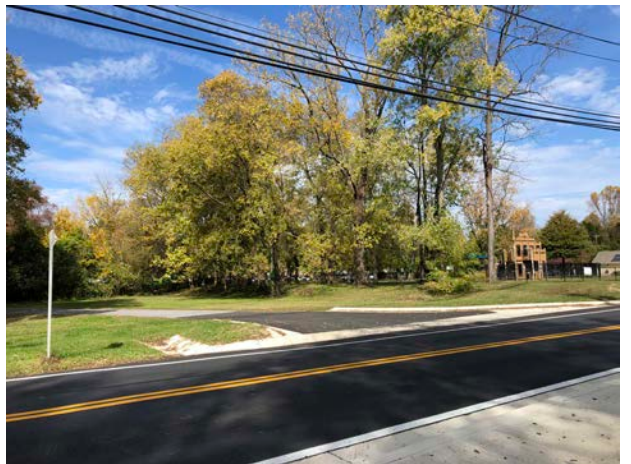
View looking north across Old Crain Highway at the Town-owned road and abandoned rail line
