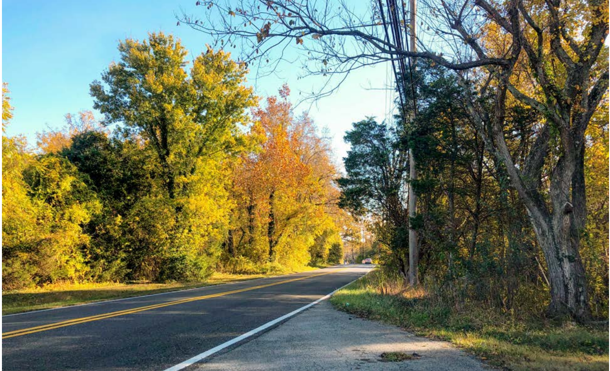
View looking east along Old Marlboro Pike from west of the abandoned rail line intersection.
