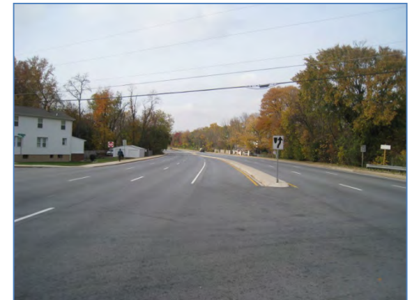
Figure 6. Un-signalized intersections lack pedestrian crossing facilities.
