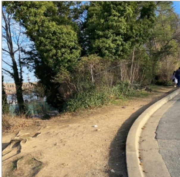
Figure 22. The east side of 18th Avenue south of Hannon Street lacks a sidewalk. (PHOTO BY TOOLE DESIGN GROUP)
