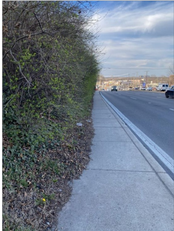
Figure 9. Vegetative overgrowth on this sidewalk at Riggs Road near University Boulevard causes a narrow walkway. (PHOTO BY TOOLE DESIGN GROUP)
