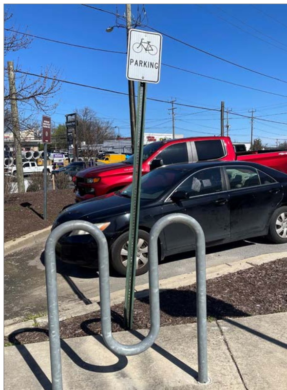
Figure 13. This inappropriate bike rack design falls short of County specifications. (PHOTO BY M-NCPPC)
