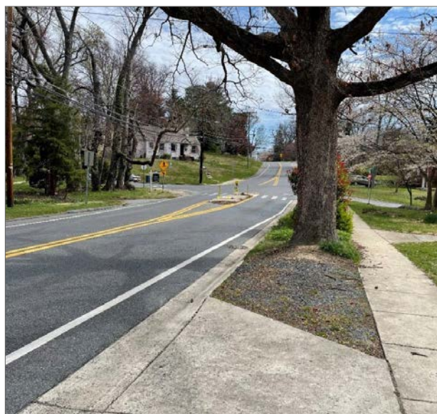
Figure 59. A pedestrian crossing island at a Franklin Avenue intersection in Silver Spring, MD. (PHOTO BY TOOLE DESIGN GROUP)
