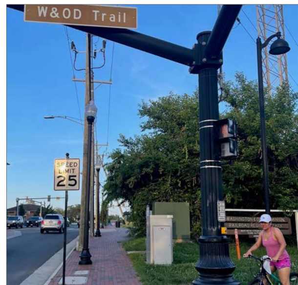
Figure 60. A mast arm-mounted street name sign improves recognition of a shared-use path intersection in Herndon, VA. (PHOTO BY M-NCPPC)
