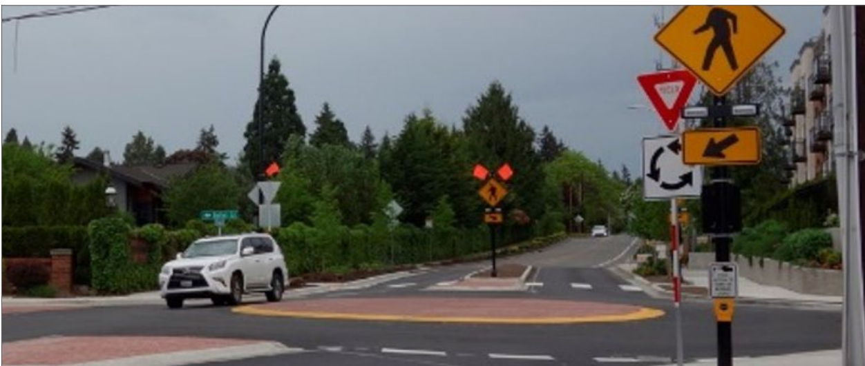
Figure 52. By comparison, construction of a mini roundabout at the Erskine/Drexel Street/18th Avenue intersection can slow motor vehicle speeds, organize traffic movement, and reduce turn conflicts. (PHOTO BY TOOLE DESIGN GROUP)
