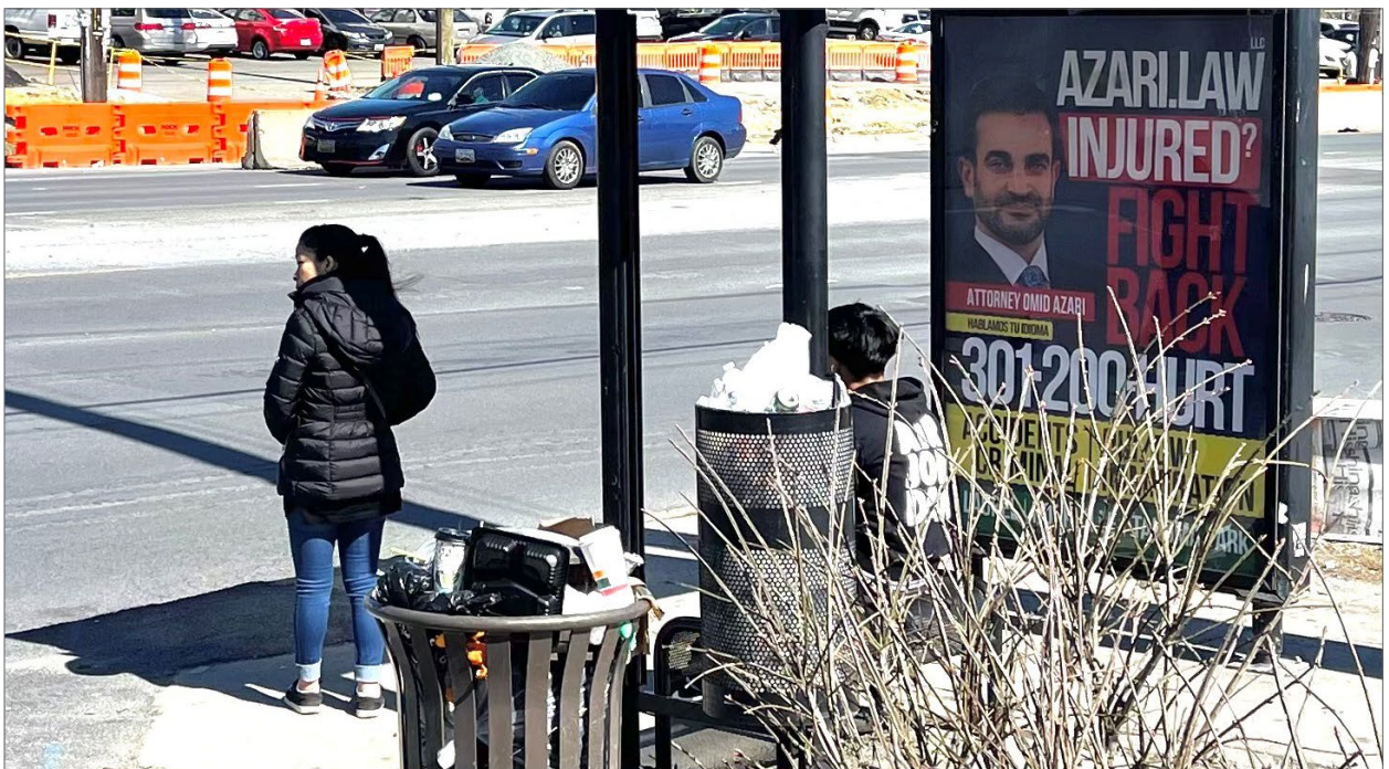
Figure 15. The only sheltered bus stop in Carole Highlands has missing glass panels and overflowing trash receptacles. (PHOTO BY M-NCPPC)
