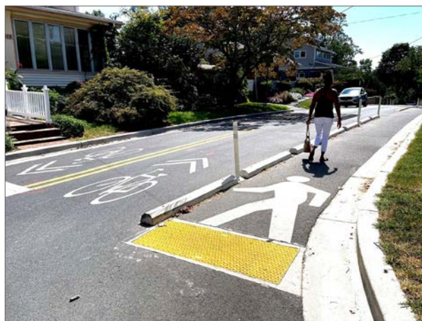
Figure 58. A protected pedestrian lane in Silver Spring directs walkers along a street without sidewalks. (PHOTO BY TOOLE DESIGN GROUP)
