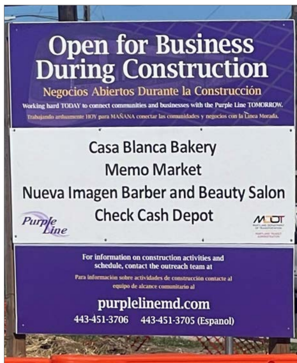
Figure 34. Purple Line construction along MD 193 (University Boulevard) has caused business disruption along the International Corridor, within and adjacent to Carole Highlands. (PHOTO BY M-NCPPC)
