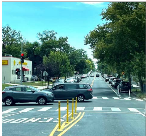
Figure 56. Flex posts shorten pedestrian crossing distances at 13th and Upshur Streets in northwest D.C. (PHOTO BY M-NCPPC)
