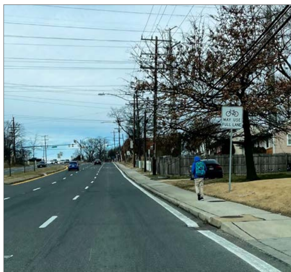
Figure 39. Median reduction presents an opportunity to convert the Riggs Road sidewalk into a shared-use path. (PHOTO BY M-NCPPC)
