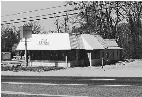
Vacant and underutilized properties provide opportunities for infill and redevelopment.
