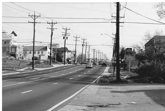
Numerous poles and inadequate pedestrian facilities project a less-than-inviting environment.
