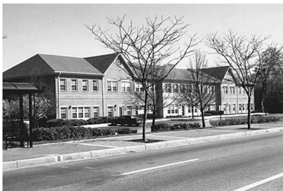
Infill commercial office development in downtown College Park partially satisfies market demand.
