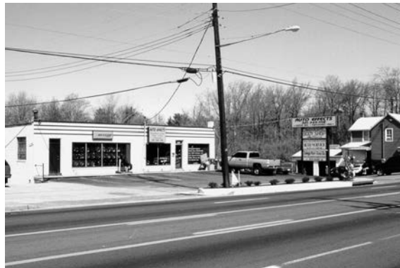
Individual curb cuts and vehicular access controls are lacking along the majority of US 1.
