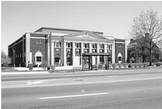
Ritchie Coliseum contributes to the academic setting of buildings facing Baltimore Avenue.
