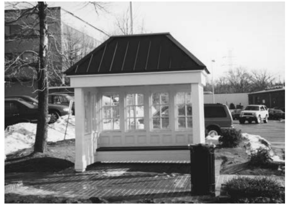
Amenities should be provided to encourage alternative modes of transportation other than single-occupant vehicle (SOV) trips.
