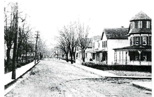
This early (circa 1910) photograph shows one of Hyattsville's streets, lined with Victorian houses.
