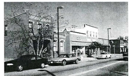
Laurel's Main Street exhibits 19th-century commercial architecture.
