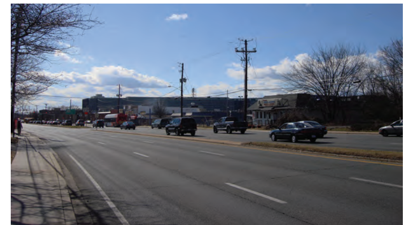
MD 458 (Silver Hill Road) runs along the top of a plateau between two watersheds and is relatively flat compared to other areas within the sector plan boundary. The U.S. Census Bureau is visible in the distance.
