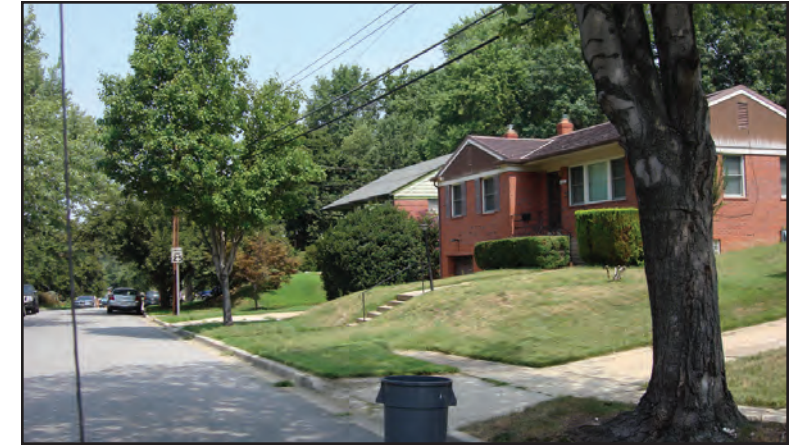
Abrupt end to the sidewalk on 25th Place in Hillcrest Heights.
