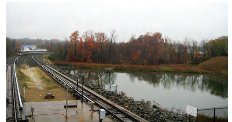
A Metrorail train on an embankment near Henson Creek rounds the curve approaching the Branch Avenue Metro Station. The pond was constructed for stormwater management.
