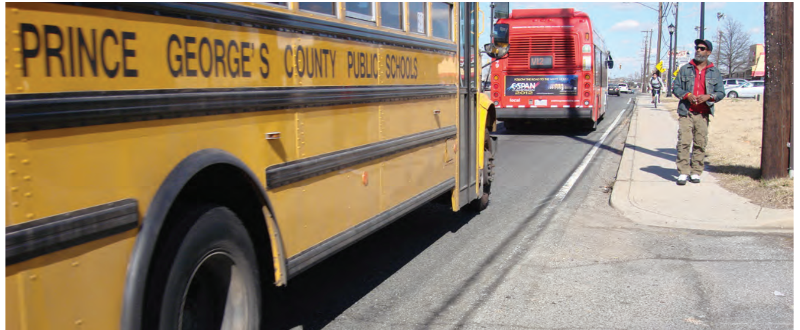
Pedestrians, bicyclists, and buses mix in a very narrow space along with the clutter of poles, lamps, and signs on the south side of Silver Hill Road.
