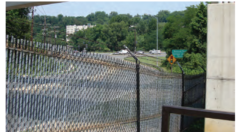
Barbed wire and a reinforced chain link fence show WMATA's determination to block an informal access point to the station from Naylor Road.
