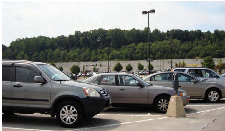
The bluff above the Southern Avenue Metro Station is 70 feet higher than the station parking lot with steep slopes.
