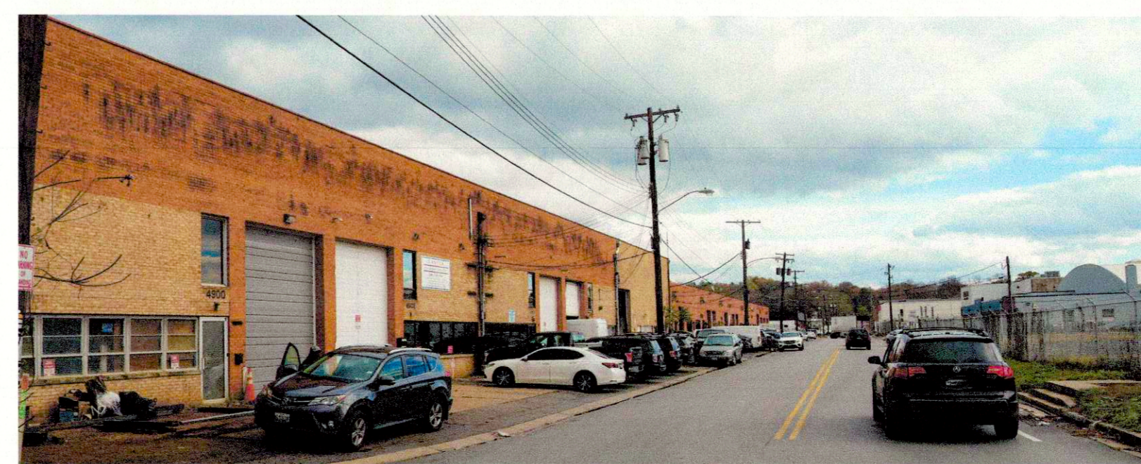
Industrial Corridor in Edmonston Source: M-NCPPC
