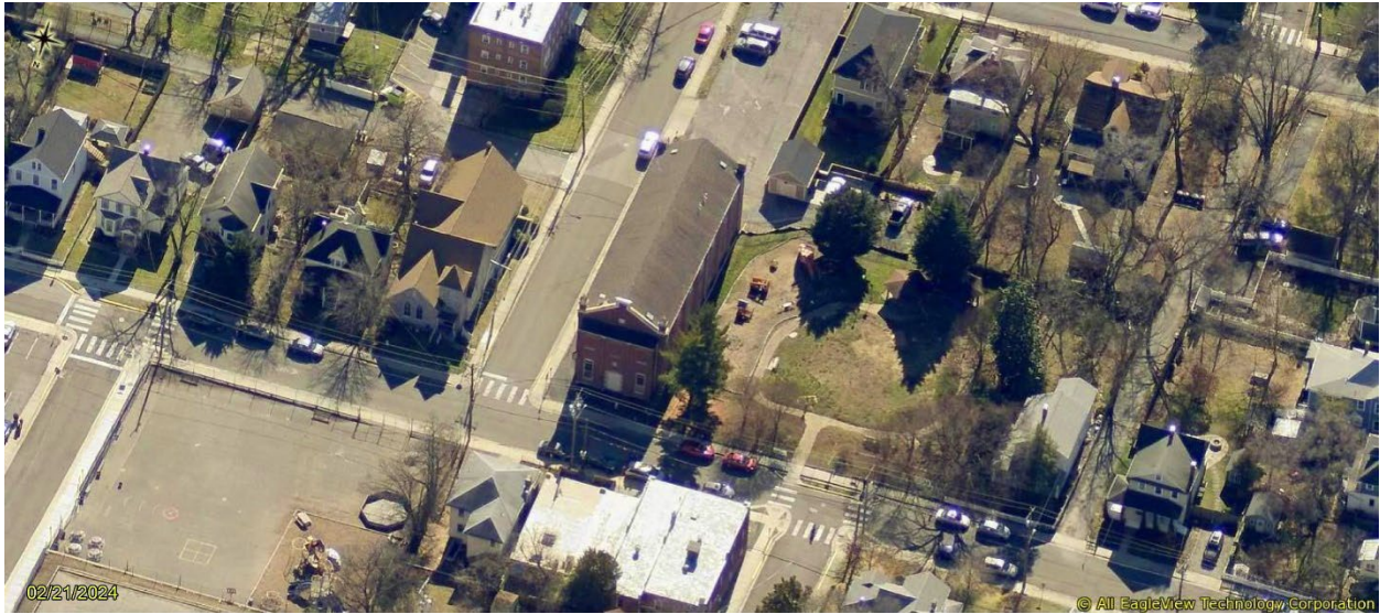
Figure 8. Bird's eye view aerial photograph of the Mount Hermon Masonic Temple, north elevation, 2024 EagleView (formerly known as Pictometry) via PGAtlas ( https://www.pgatlas.com/ )
