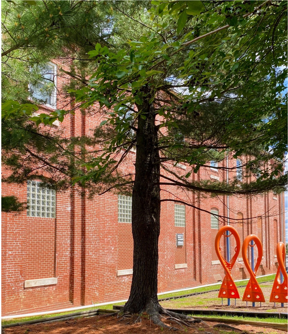
Mount Hermon Masonic Temple, partial view of west elevation, May 11, 2024.
