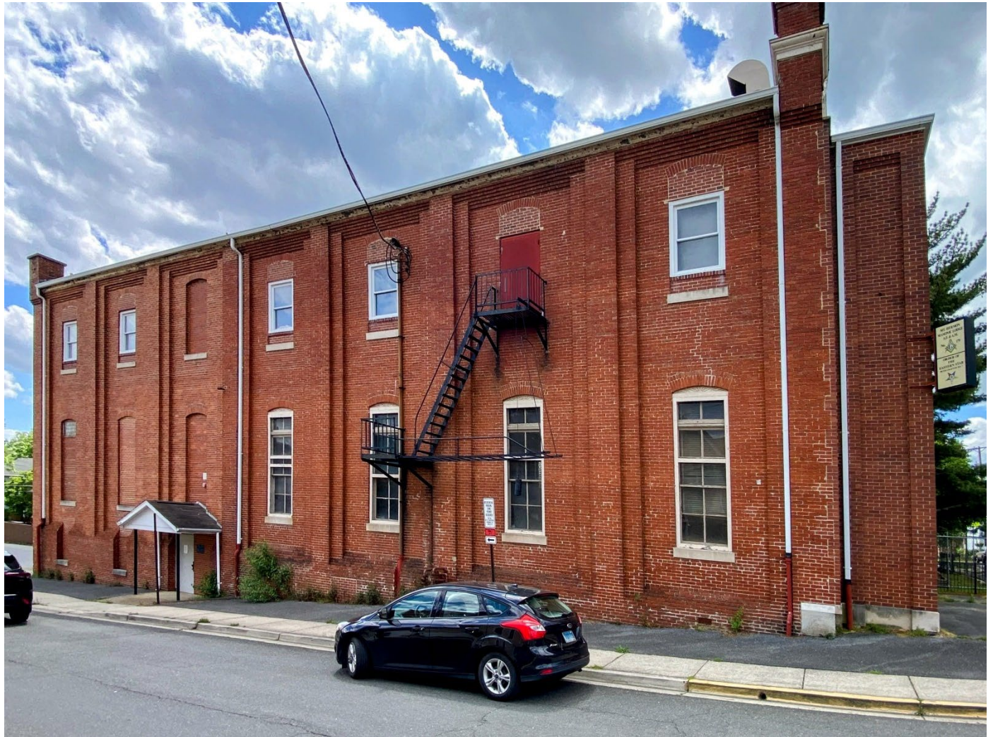
Mount Harmon Lodge Masonic Temple, east elevation, May 11, 2024.
