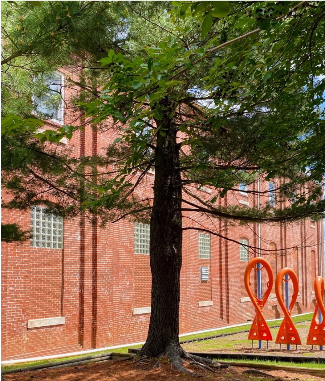
Figure 15. Mount Hermon Masonic Temple, partial view of west elevation, May 11, 2024
