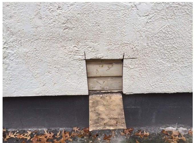
East elevation. Portion of stucco removed to show original drop siding underneath, which will be restored.
