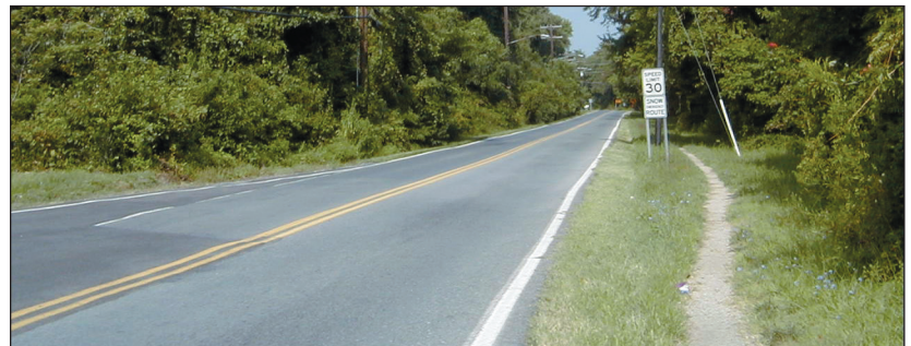
Existing facilities for pedestrians and bicyclists are fragmented or missing in many areas. Continuous sidewalks and designated bike lanes are recommended.
