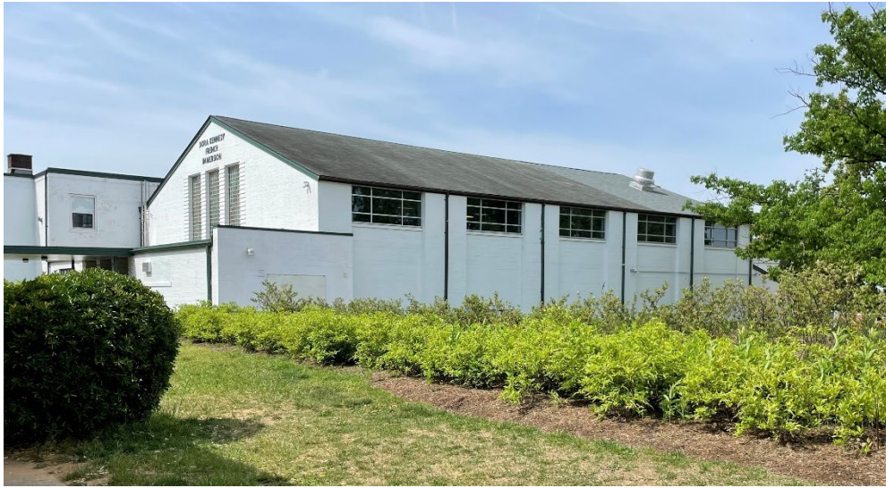
Figure 7. Greenbelt Middle School, 1953 gymnasium addition, north and east elevations, May 2024.
