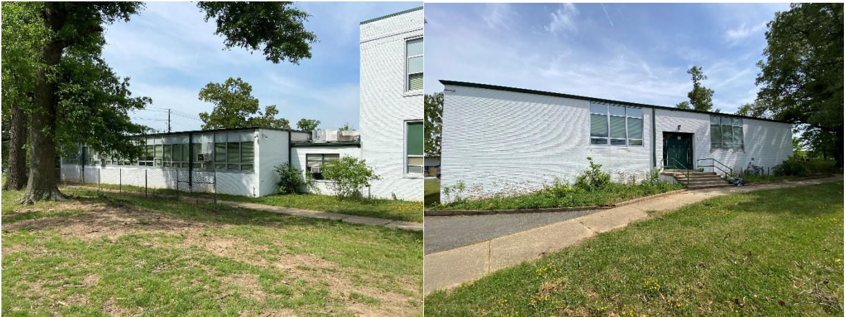
Figure 8. Greenbelt Middle School, 1963 addition, east and south elevations, May 2024.
