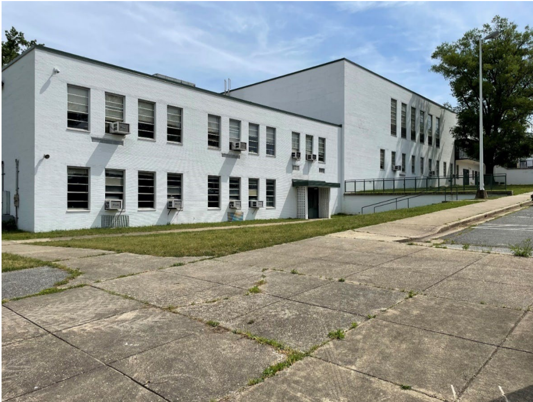
Figure 10. Greenbelt Middle School 1969 addition, south elevation, May 2024.
