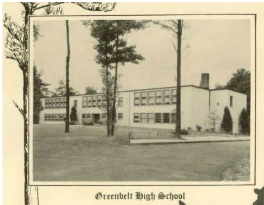
Figure 12. Photo of 1938 building from the 1940 Pylon (Greenbelt High School Yearbook).
