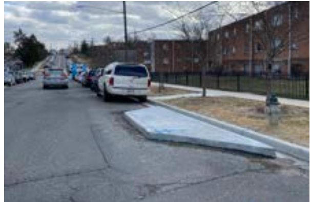
Recently installed curb extension on 15th Avenue.
