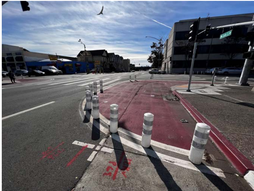
Figure A14. Curb Bulb Outs
