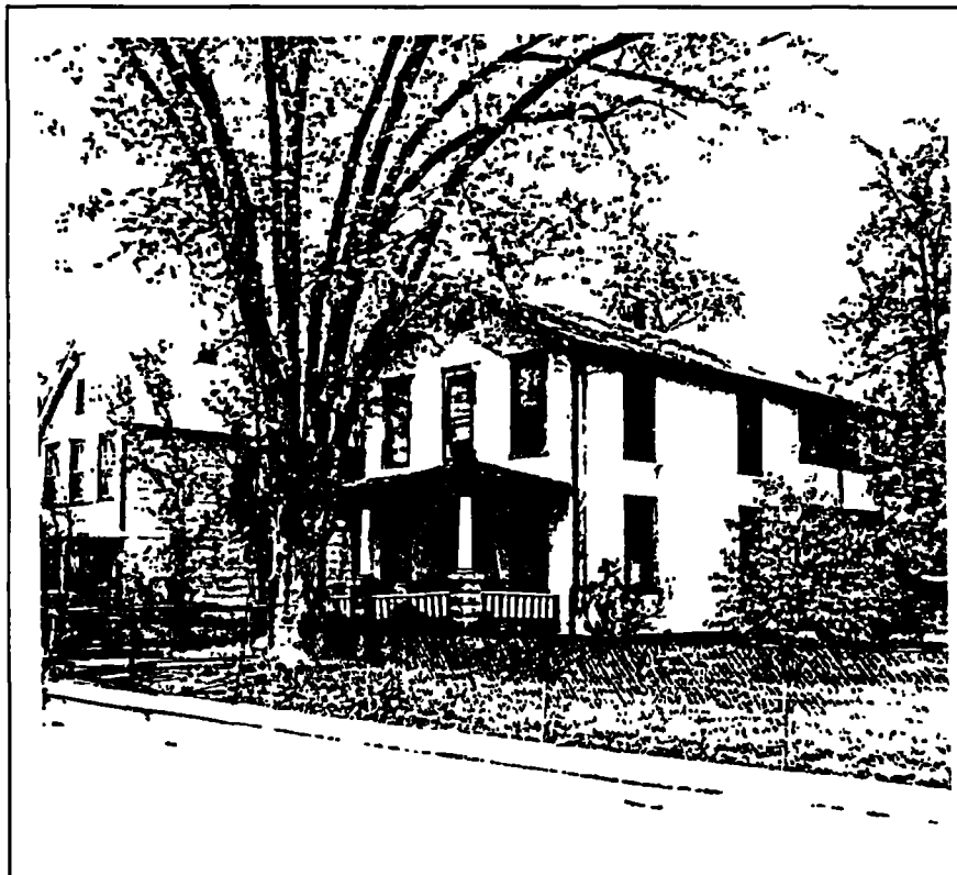
Figure 29 - The A. A. Henning House (right): Block 9, lot 16, Brentwood subdivision 3606 Varnum (originally Evans) Street - front-gabled frame (later stuccoed) dwelling built in 1903.
