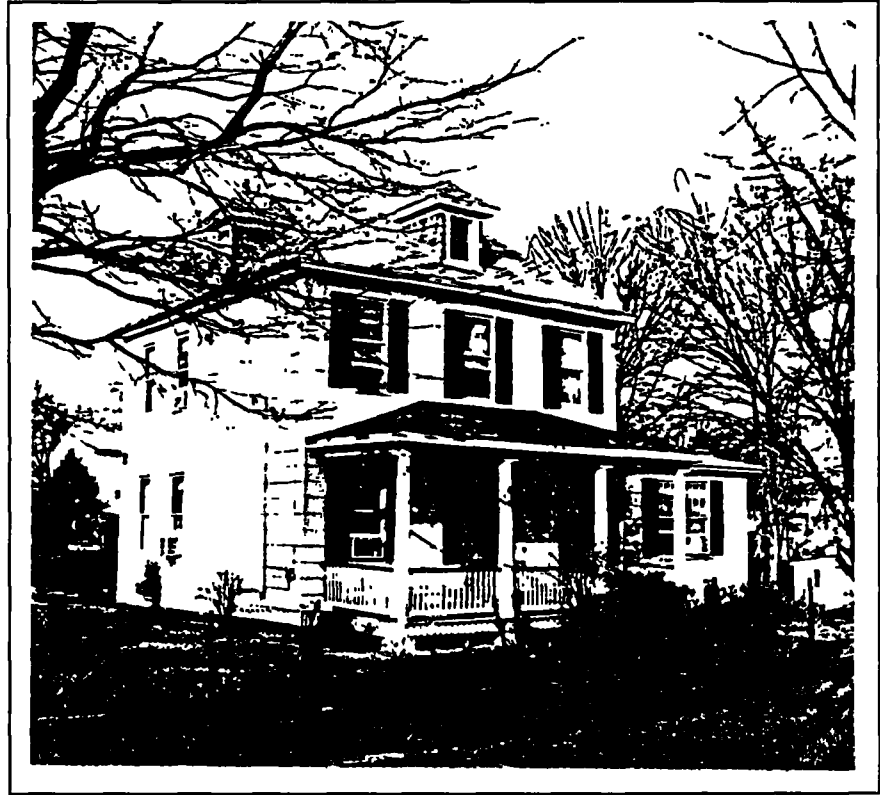
Figure 24 - The John Pribula House: Block 3, lot 6, Brentwood subdivision 3500 Taylor (originally Baker) Street American Foursquare frame dwelling built by 1905.
