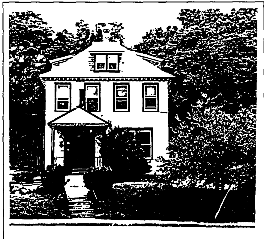
Figure 25 - The Winter Gigous House: Block 18, lot 5, Holladay Company subdivision - 3900 Rhode Island (originally Highland) Avenue - Colonial Revival Foursquare frame dwelling built in 1905.
