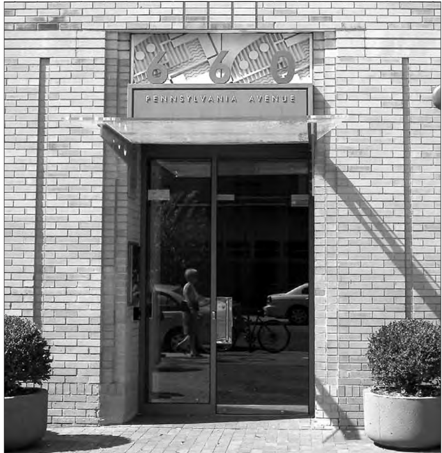
Highlight entrances by adding awnings, a legible street number, facade detailing, and plantings so that visitors may find them.
