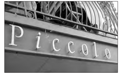
These are two examples of pin letters, signage attached to the face of a building by pins.
