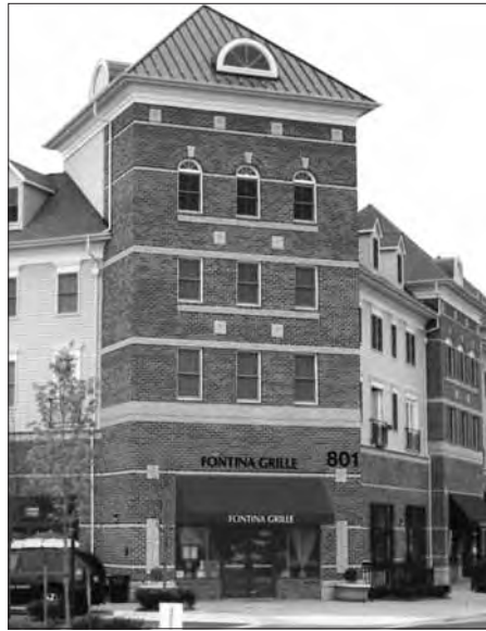
Buildings at street intersections orient doors, windows, and architectural details toward the corner to maximize neighborly interaction and economic potential.
