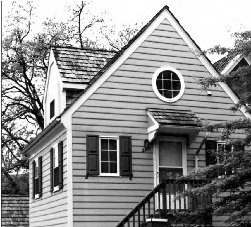
The windows on this second story granny flat are well articulated with frames, sills, and correctly proportioned shutters with shutter hooks.
