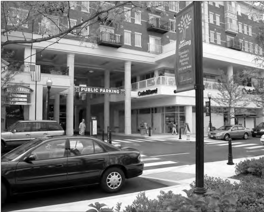
This structured parking is highly visible, attractive, and wrapped by commercial development.
