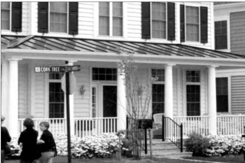
Usable porches and balconies enable residents to meet their neighbors and allow natural surveillance of the street.
