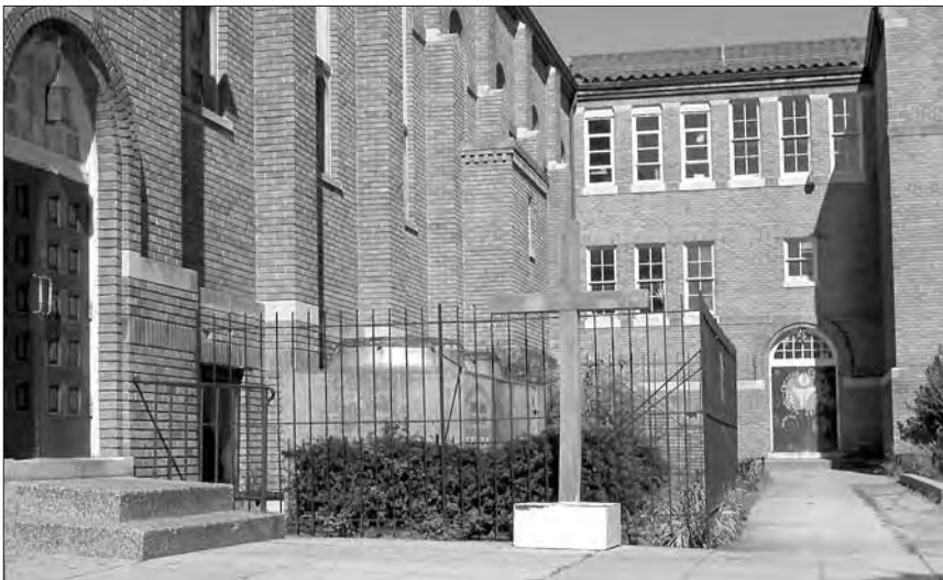
This fence and landscaping inadequately screen the mechanical equipment.
