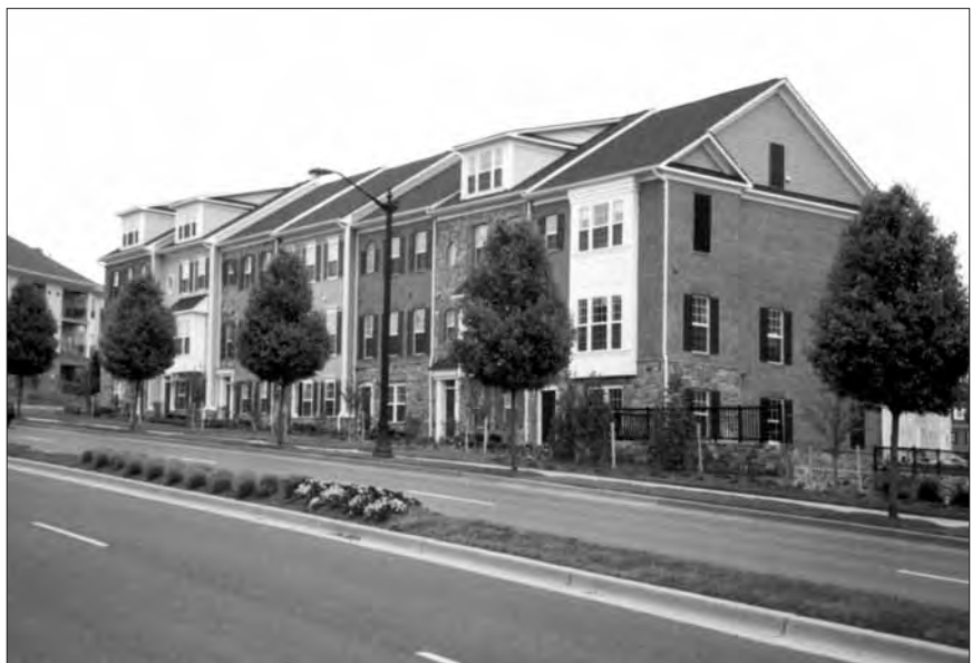
This residential building is divided into vertical bays that alternate materials so that each unit "reads" as a separate structure.
