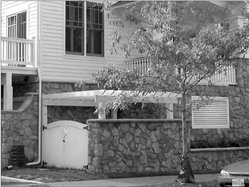
Screen trash and dumpster areas with structures that are compatible with the main building.
