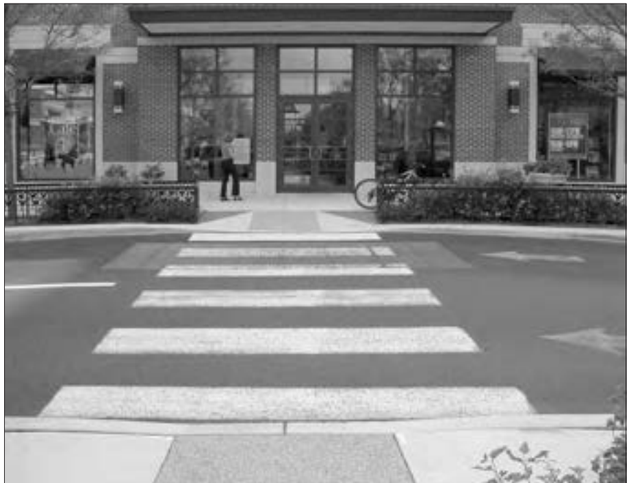
Design pedestrian crossings using the shortest crossing distance (at a right angle to the street direction) and access ramps to make streets safer and accessible to all users.
