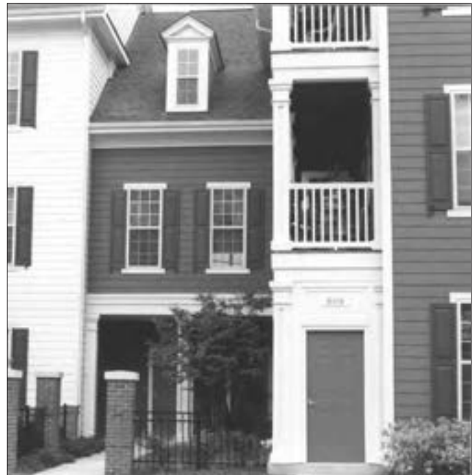
Build in natural surveillance and increase safety by connecting residences to streets and alleys through windows, balconies, porches, stoops and gardens.
