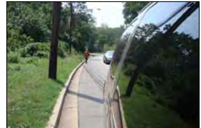
A pedestrian is forced to walk on the road along 23rd Parkway.
