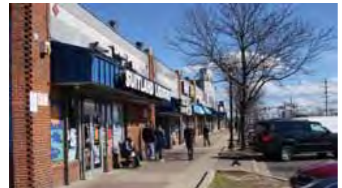
The Suitland Corners block received a façade improvement in the late 1990s funded by the State of Maryland.
