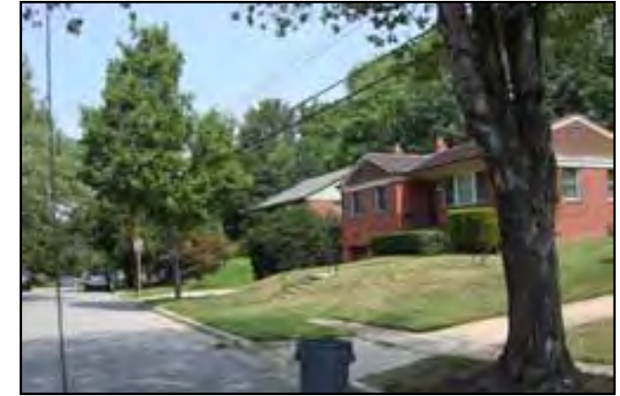
Abrupt end to the sidewalk on 25th Place in Hillcrest Heights.
