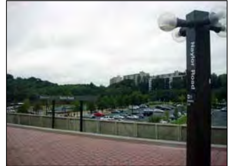
View from the elevated station platform showing station parking and apartment buildings on a low bluff south of the station.
