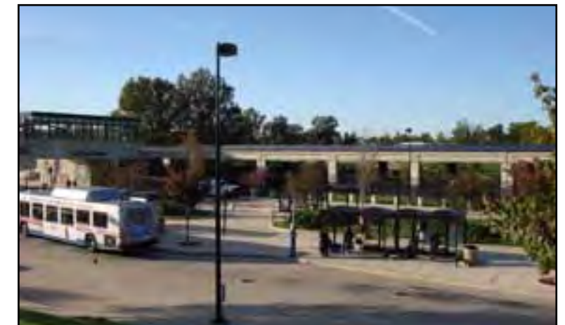
Suitland station also serves as a bus hub for bus to rail and bus to bus transfers.
