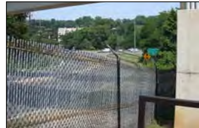
Barbed wire and a reinforced chain link fence show WMATA's determination to block an informal access point to the station from Naylor Road.
