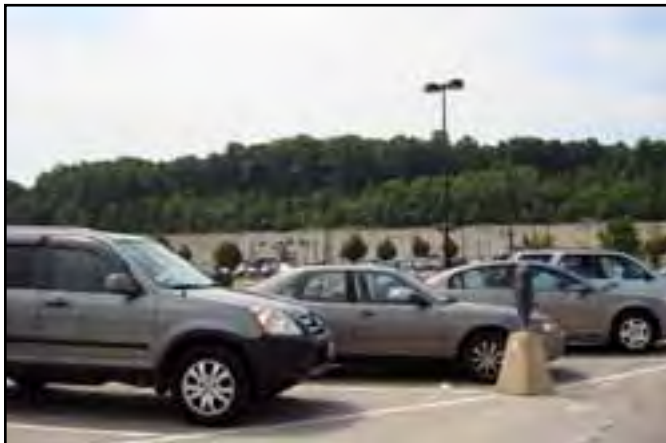
The bluff above the Southern Avenue Metro Station is 70 feet higher than the station parking lot, with steep slopes.
