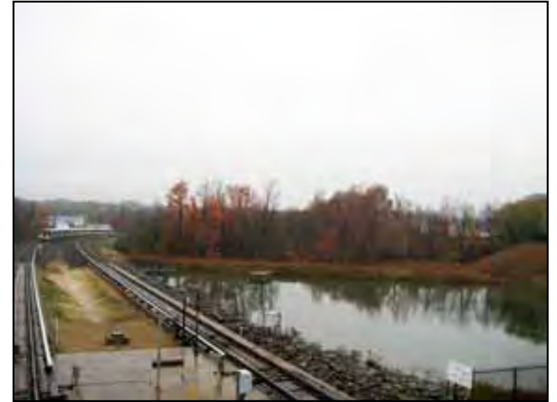
A Metrorail train on an embankment near Henson Creek rounds the curve approaching the Branch Avenue station. The pond is an artificial construction to manage stormwater.
