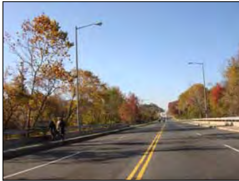
The bridge over the Oxon Run stream provides pedestrian access to the Southern Avenue Metro Station. In the distance the land rises above the stream valley floor.
