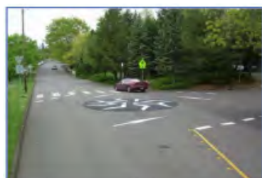
Photo 3. Potential improvement: Low-profile traffic circle.
