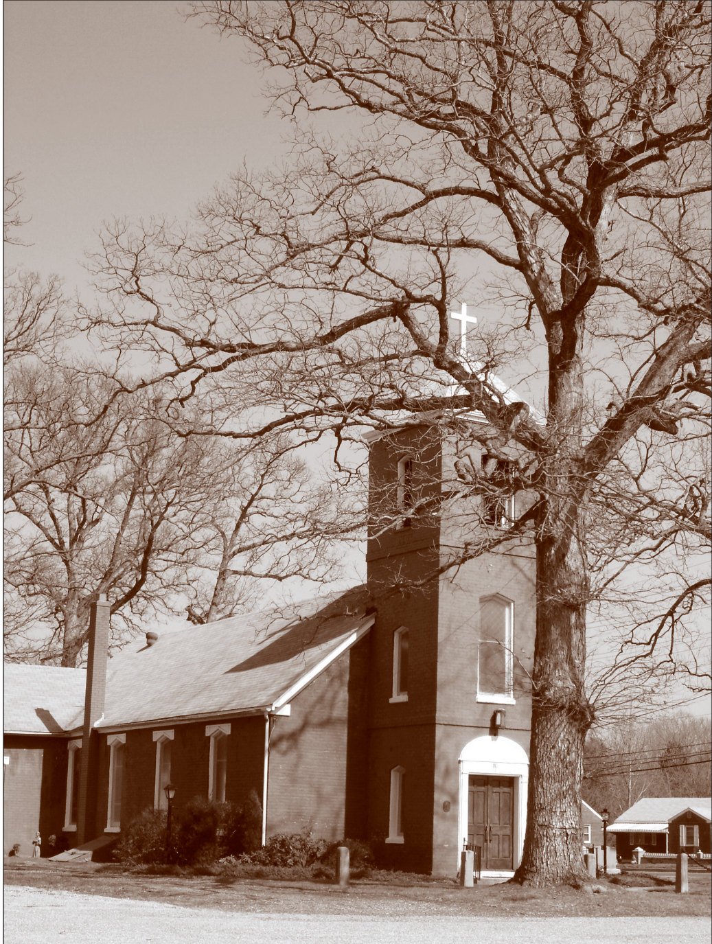
County Historic Site 76A-004, the St. Barnabas Episcopal Church.
