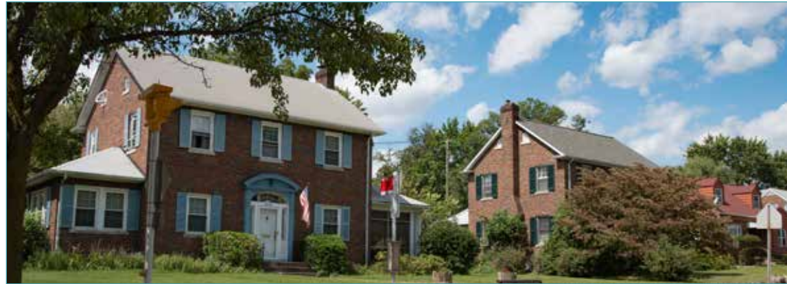
The Town of Cheverly contains a variety of buildings constructed between 1920 and the 1950s.
