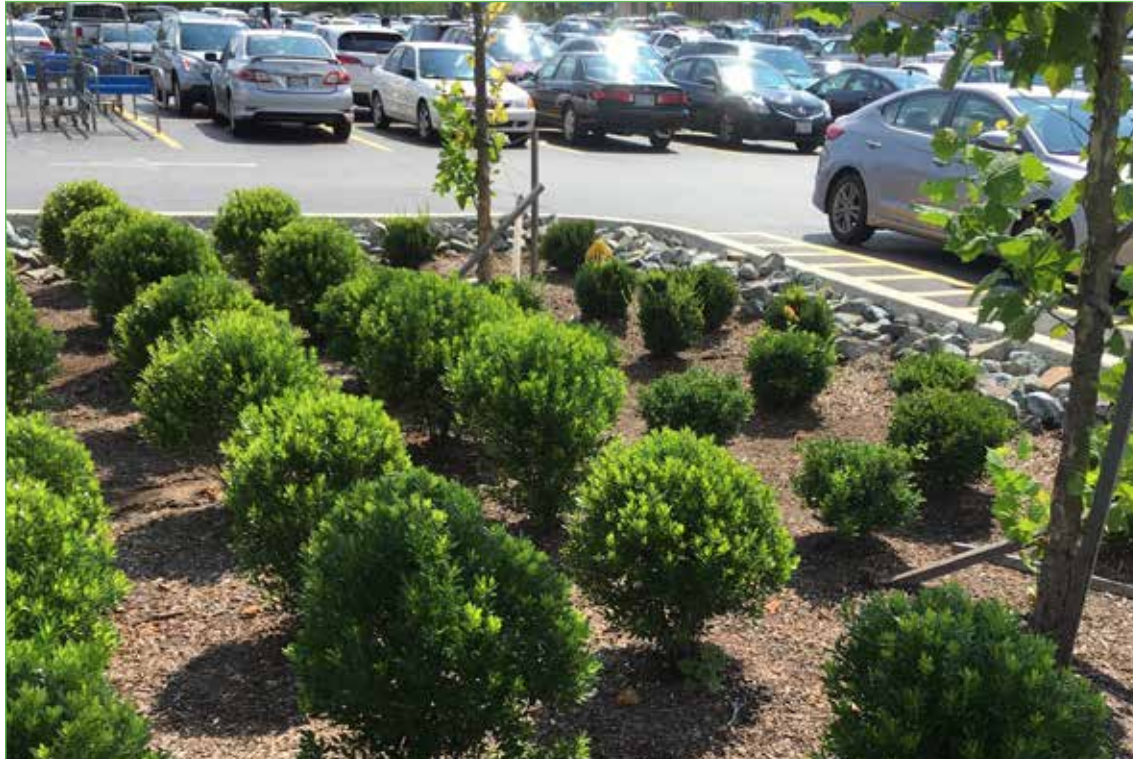
Parking lot bioretention provides shade as well as stormwater management.
