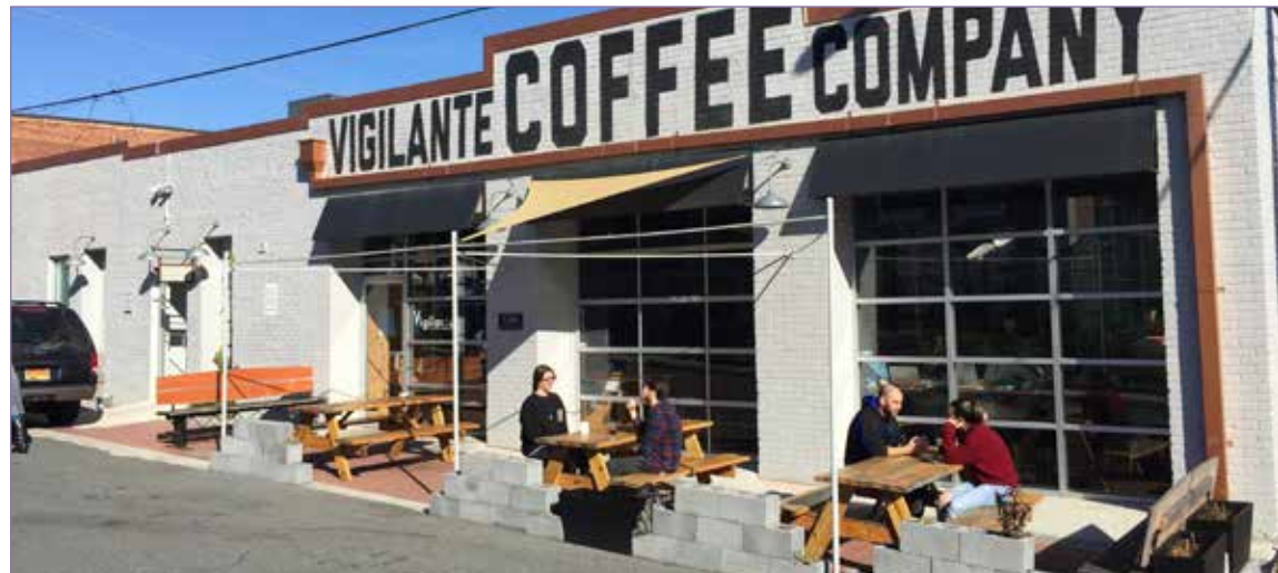
Vigilante Coffee in Hyattsville is located in a building formerly used for auto servicing
