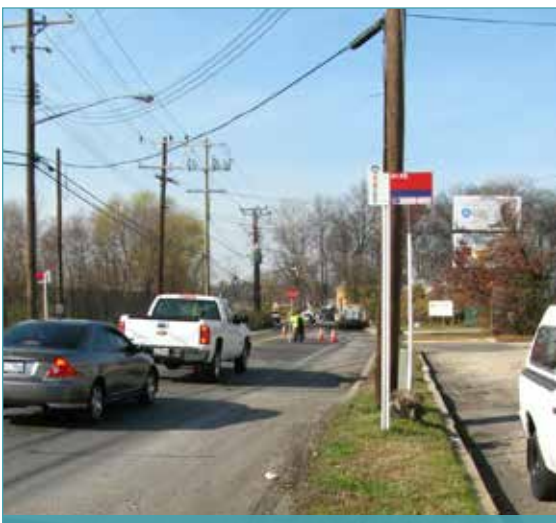
Many bus stops are poorly located and lack ADA-accessible landing pads.
