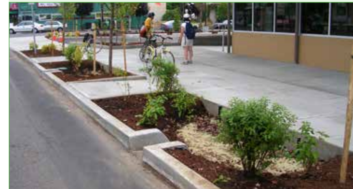
Bioswales are valuable interventions to treat runoff along linear facilities, such as roads, parking lots and buildings.
