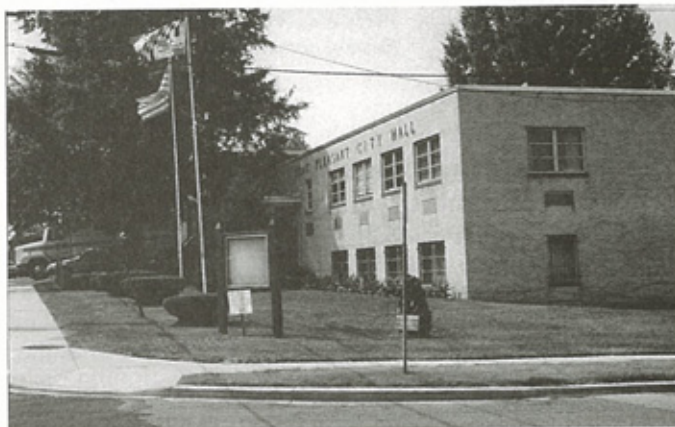
Public uses increase the viability of the town center as a community focal point.
