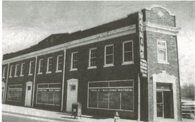
The Old Town Commercial Area can complement the Metro Town Center.
