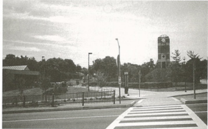
Recent pedestrian safety improvements on MD 214 improve access to the station.
