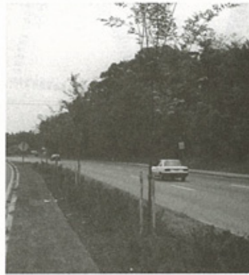
Plantings in the MD 214 median create interest, color and continuity along this busy roadway.
