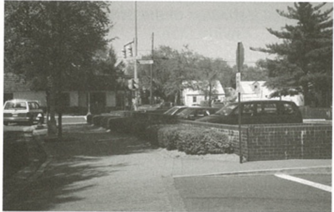
Low masonry walls and evergreen shrubs are recommended to screen parked cars from the roadway.
