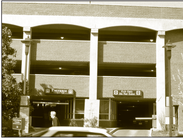
One or more attractive parking garages may at some time be needed to support the Arts District.
