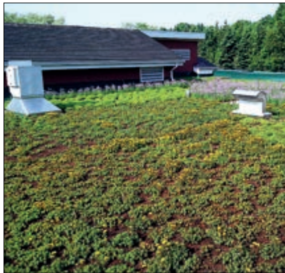
Building with Green Roof
