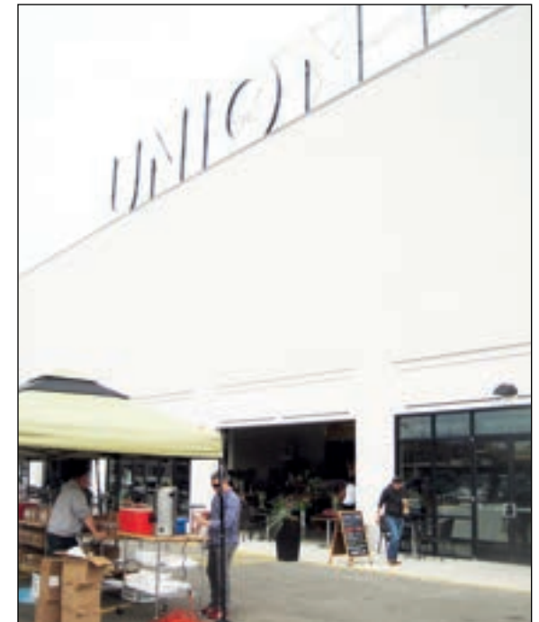
Adaptive Reuse of Industrial Building for Union Market
