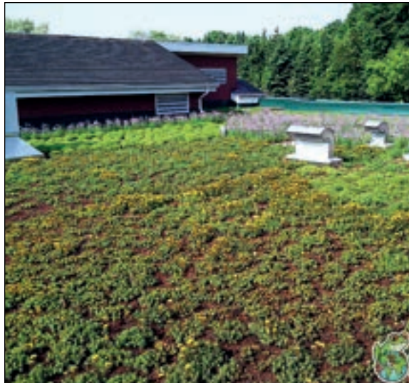
Industrial Building with Green Roof
