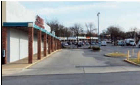
Existing Entrance to the Center from Dodge Park Road
