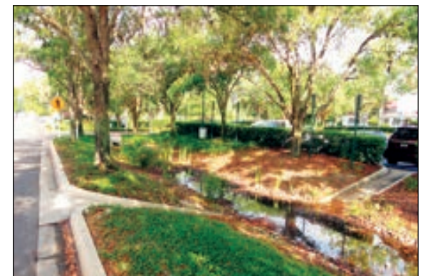
Parking Lot with Landscaped Island for Stormwater
