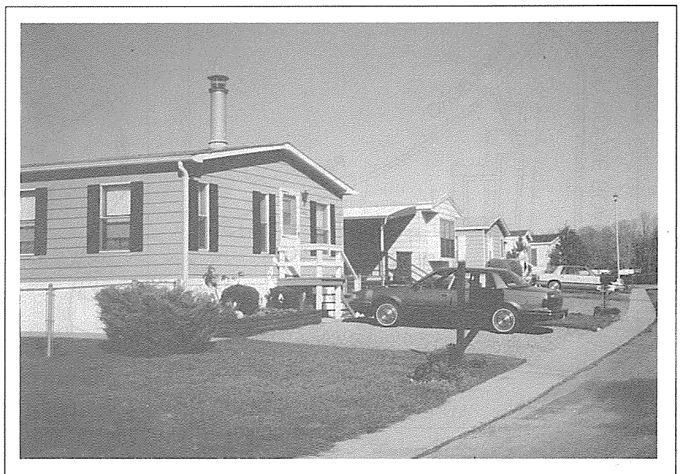
Street scene in the Flower Village Mobile Home Park showing the neatly landscaped units and off-street parking that make this a model community.
