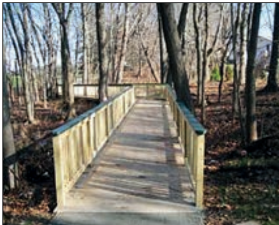
Walkway through an Environmentally Sensitive Area
