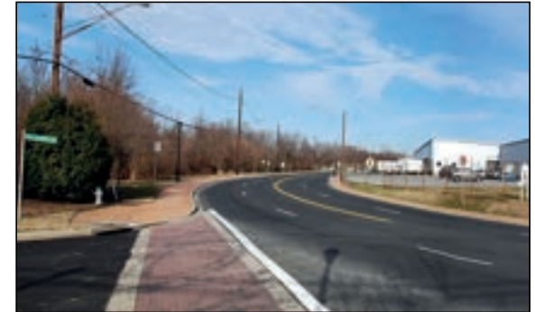
Existing Pennsy Drive Leading to Metro Station
