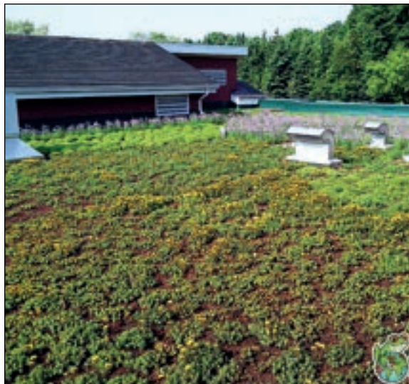
Industrial Building with Green Roof
