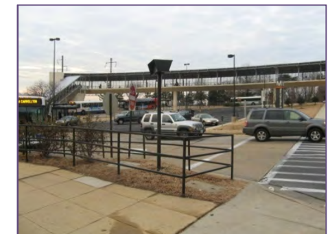
Existing pedestrian bridge linking IRS Building and New Carrollton Transit Station
