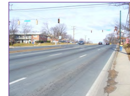
Narrow sidewalk along Riggs Road facing east
