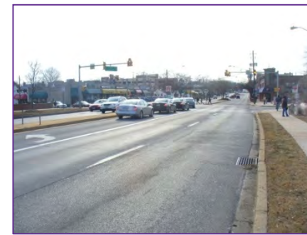
Baltimore Avenue (US 1) at College Avenue intersection facing south
