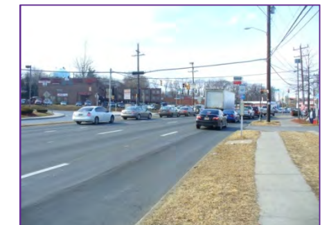
University Boulevard (MD 193) at Riggs Road intersection facing west
