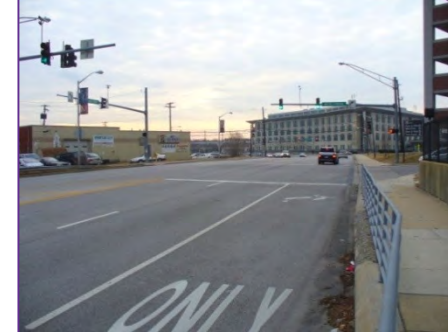
Paint Branch parkway at Metro Parking intersection facing south
