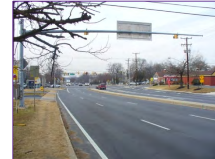
East-West Highway (MD 410) east of Kenilworth Avenue (MD 201) facing east
