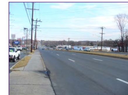
University Boulevard (MD 193) facing west
