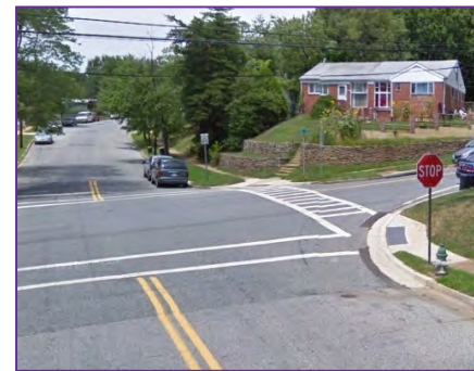
Flintridge Drive at 70 th Place intersection facing north
