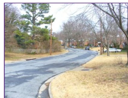
Sidewalk not provided along portions of 15th Avenue
