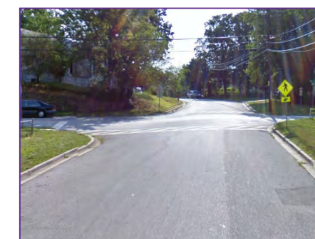
Patterson Street at 67 th Avenue intersection facing east
