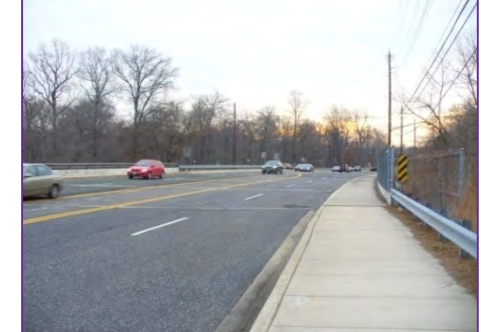
Paint Branch Parkway over the Paint Branch facing east
