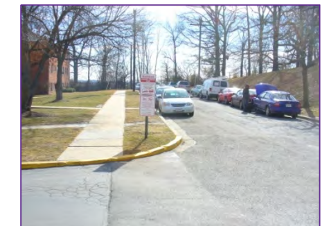
Sidewalk ramp not provided along Guilford Road facing west
