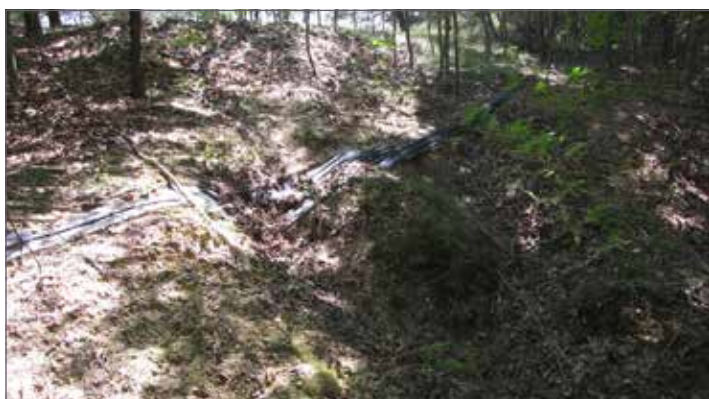
Figure 20. Breached silt fencing allows erosion of sand and gravel from closed mine into nearby stream.
