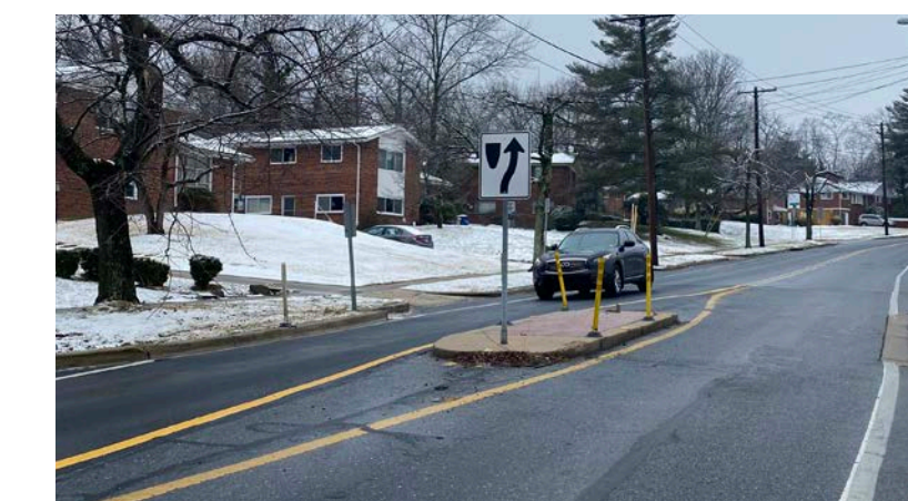
Concrete Spot Median Island
