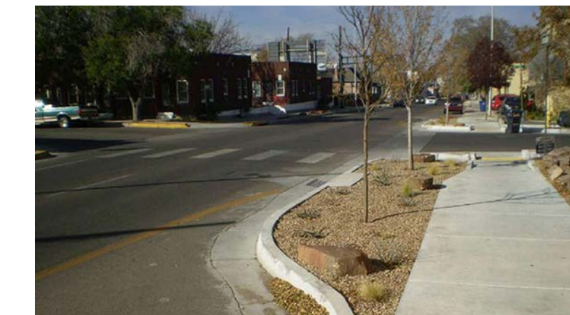
Curb Extension at Intersection Image Credit: James Barrera
