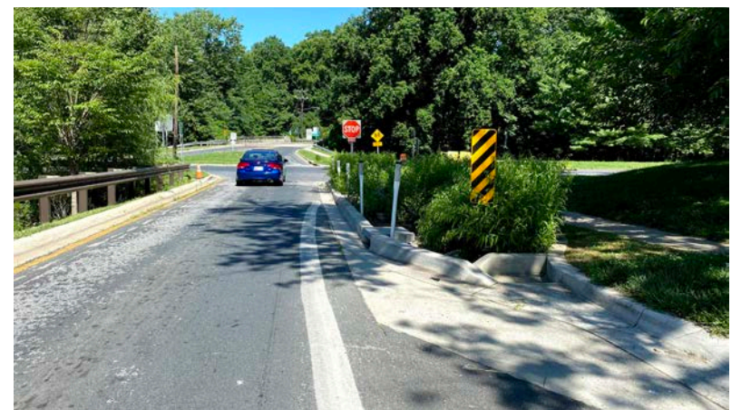
Stormwater Swale as part of Curb Extension
