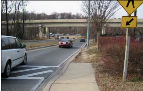
A sidewalk abruptly ends on Naylor Road. While there is a sidewalk on the other side of the road, it forces pedestrians to cross.
