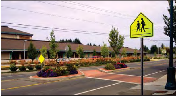
Raised Median Islands/Pedestrian Refuge Area $4,000 - $30,000 per crossing Provides a protected area in the middle of a crosswalk for pedestrians to stop while crossing street.
