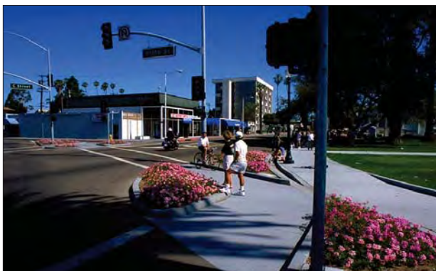
Reduced Curb Radii $5,000 - $30,000 per corner Reconstructing a street corner with a smaller radius to reduce vehicle turning speeds.
