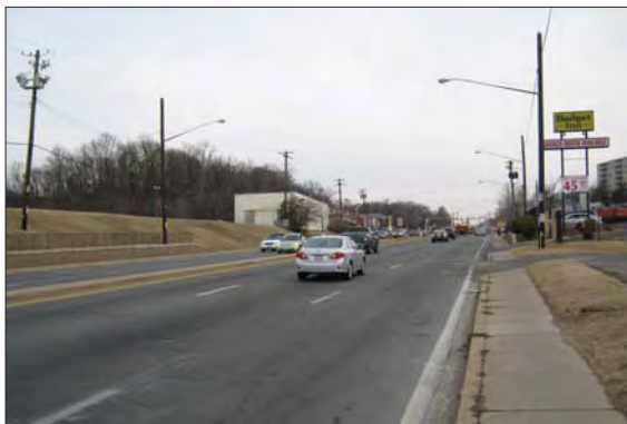
The width of the sidewalk on Branch Avenue (MD 5) frequently changes, with several narrow sections that are uncomfortable for pedestrians.
