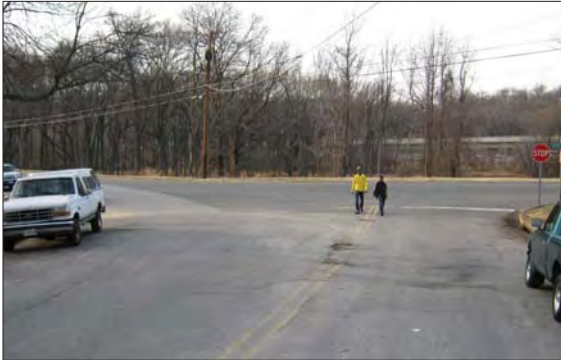
The intersection of Oxon Run Drive/Oxon Park Street is excessively large and encourages fast turning movements. Tightening this intersection would calm traffic and reduce pedestrian crossing distance.
