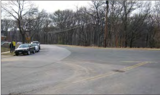
The intersection of Oxon Run Drive/28th Parkway has a large turning radius which permits vehicles to turn while maintaining high speeds.
