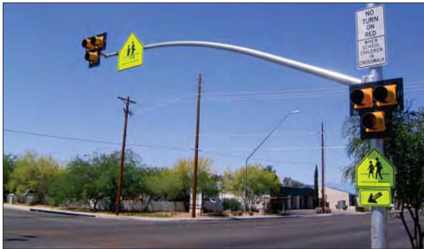
Pedestrian Hybrid Signal (HAWK) $50,000 - $75,000 per crossing Pedestrian activated signal, unlit when not in use, begins with a yellow light alerting drivers to slow, and then a solid red light requires drivers to stop while pedestrians have the right-of-way to cross the street. The example shown is at Georgia Avenue and Hemlock Street.
