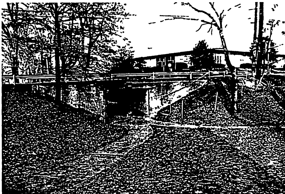
Figure 5 - Pedestrian Underpass, Crescent Road at Greenbelt Library
