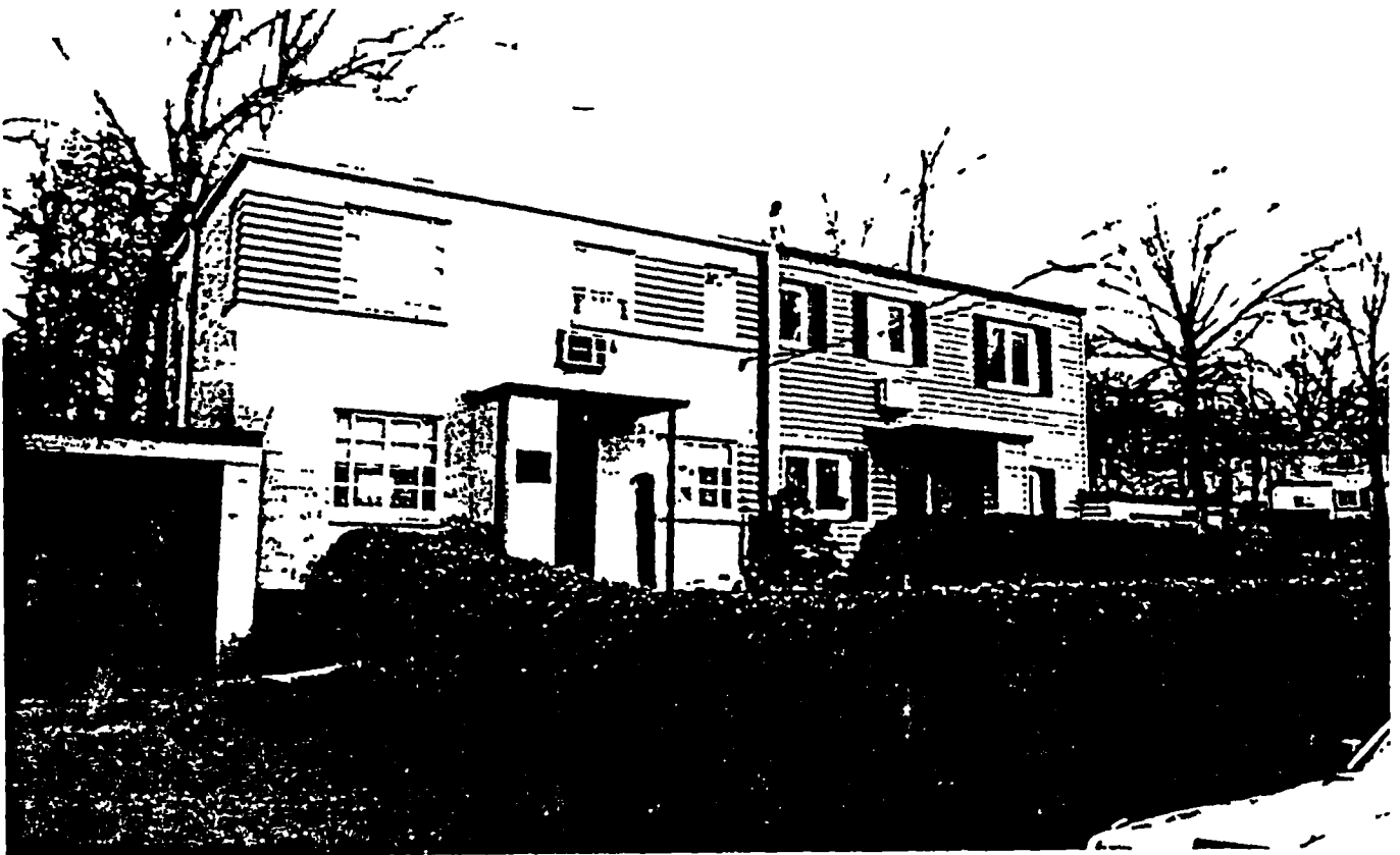
Figure 8 - Window Treatments - Original windows at left; replacements at right, Crescent Road at Westway
