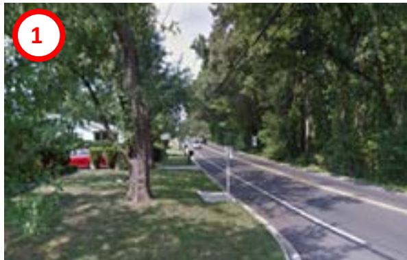
Ritchie Road northbound bus stop
