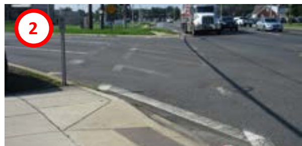
Crosswalk across east leg
