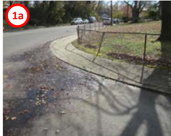
Sidewalk on southwest corner of intersection
