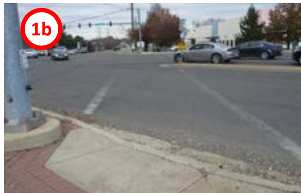
Crosswalk on east leg
