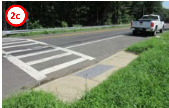
Ramp at north leg of intersection
