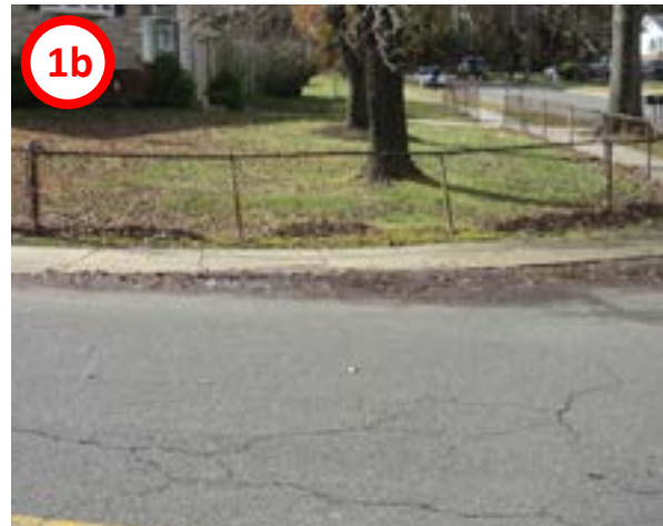
Sidewalk on southwest corner of intersection
