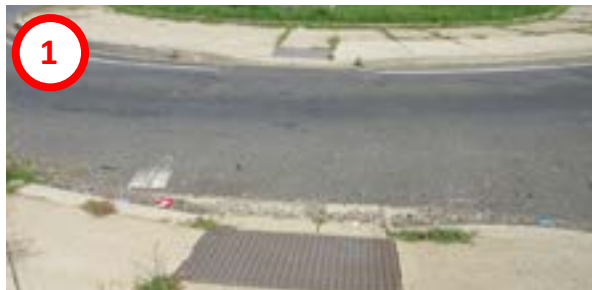
Southbound right-turn, channelized lane
