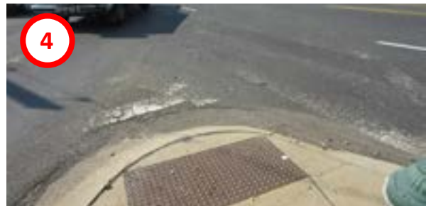
Crosswalk across west leg
