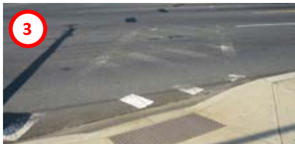
Crosswalk across north leg
