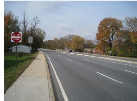
Figure 3. Sidewalks next to the roadway with few pedestrian-friendly features limit pedestrian safety and comfort.
