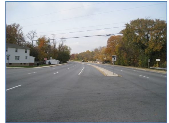
Figure 6. Un-signalized intersections lack pedestrian crossing facilities.
