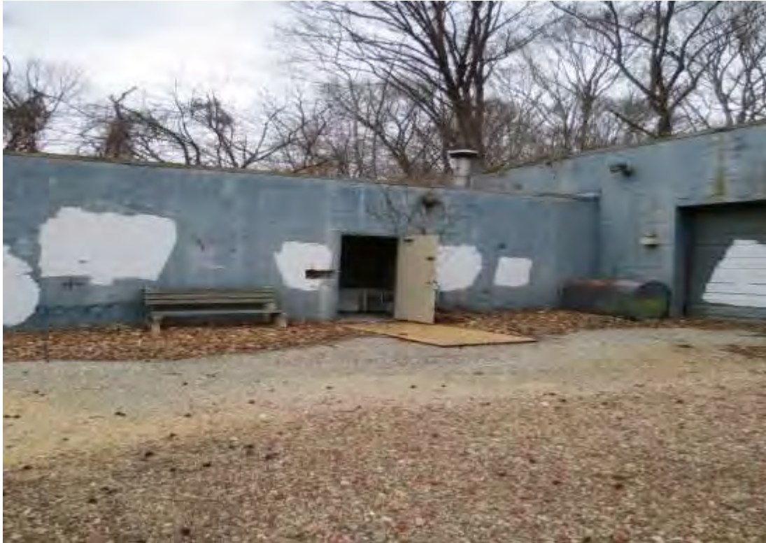
Unsecured maintenance building.
