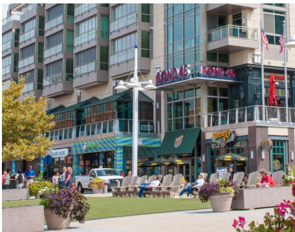
National Harbor Waterfront, retail development is oriented around pedestrian amenities, walkability, and interaction.
