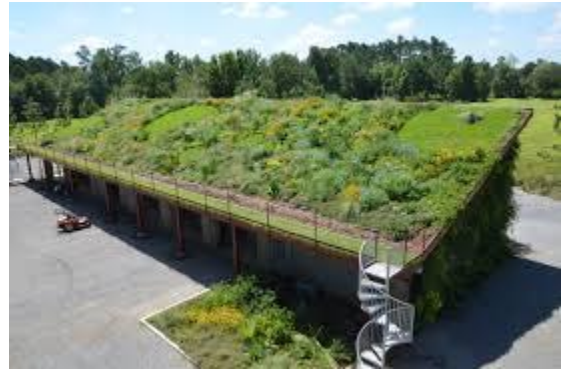
Figure 20. A rural green roof (Moore Farm, 2019)
