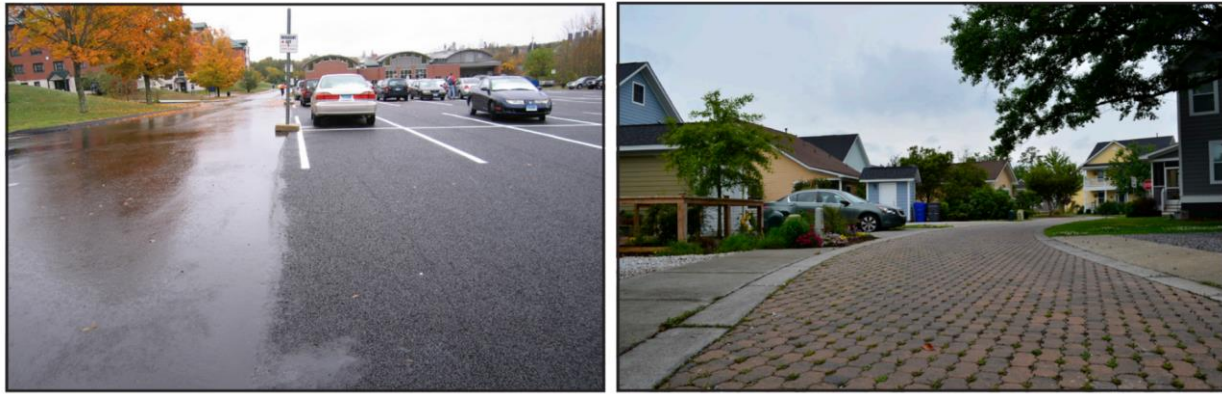
Figure 15. Permeable concrete (left) and permeable pavers (right) (NOAA, 2015)
