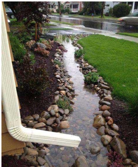
Figure 17. Disconnected downspout (Brown, 2019)
