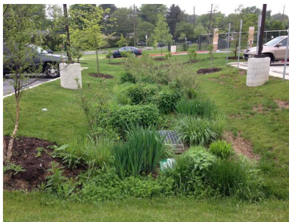
Figure 19. A rain garden (Montgomery County Government, 2019)
