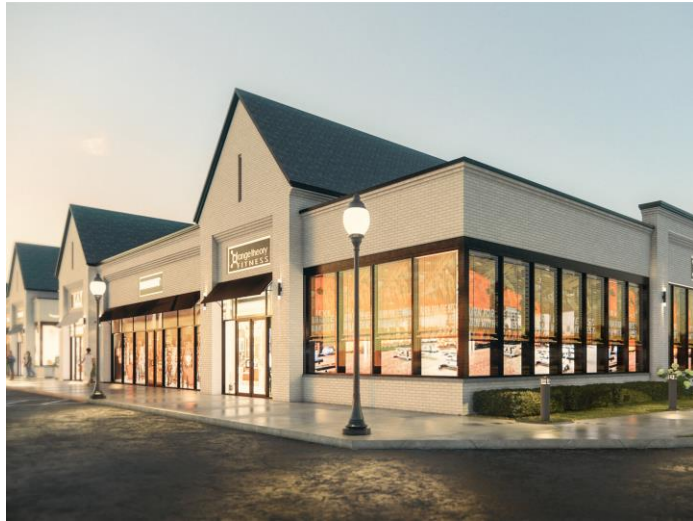
Shopping Plaza Retail (Redevelopment): Redevelopment of aging strip retail with focus on vibrancy and reference to historic village.
