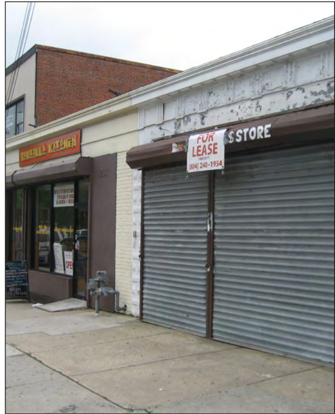
EXAMPLE OF PROHIBITED SOLID ROLL GATES.
