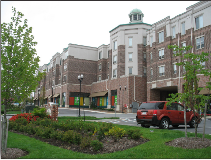
Multifamily development with retail on lower level at Trebeca at Camp Springs
