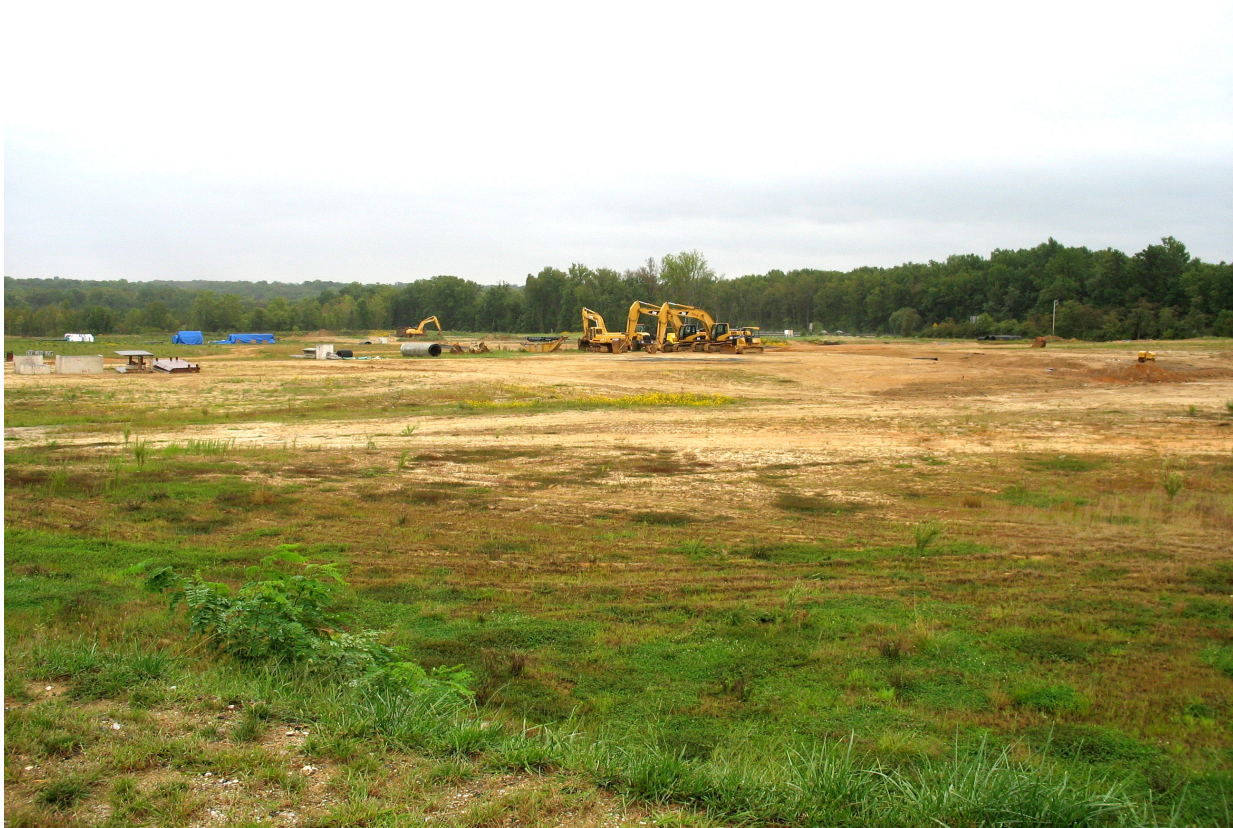
Continuing construction at Melford in Bowie
