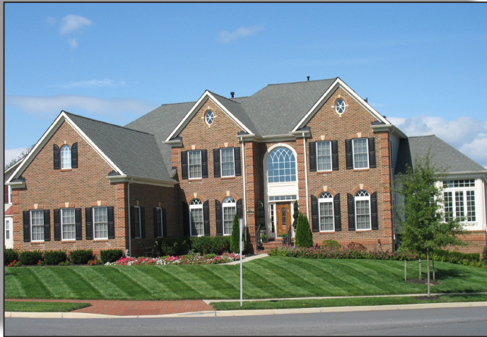
Typical single-family home at Beech Tree
