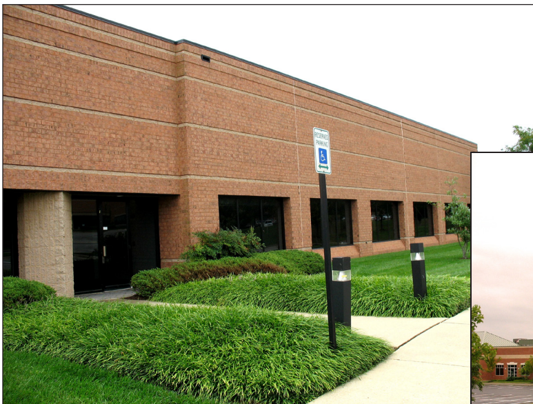
Office building at Konterra Business Center
