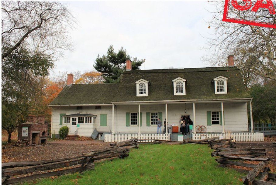
Southwest (front) elevation from Main Street, looking northeast.
